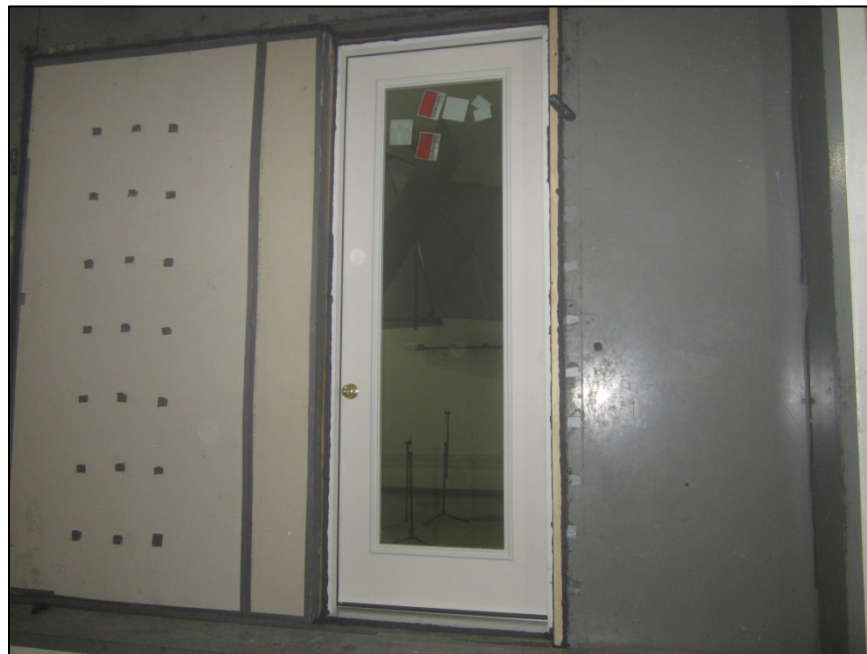
Source Room View of Installed Specimen
